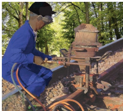
Figure 3.11 Thermit process for joining railway tracks
